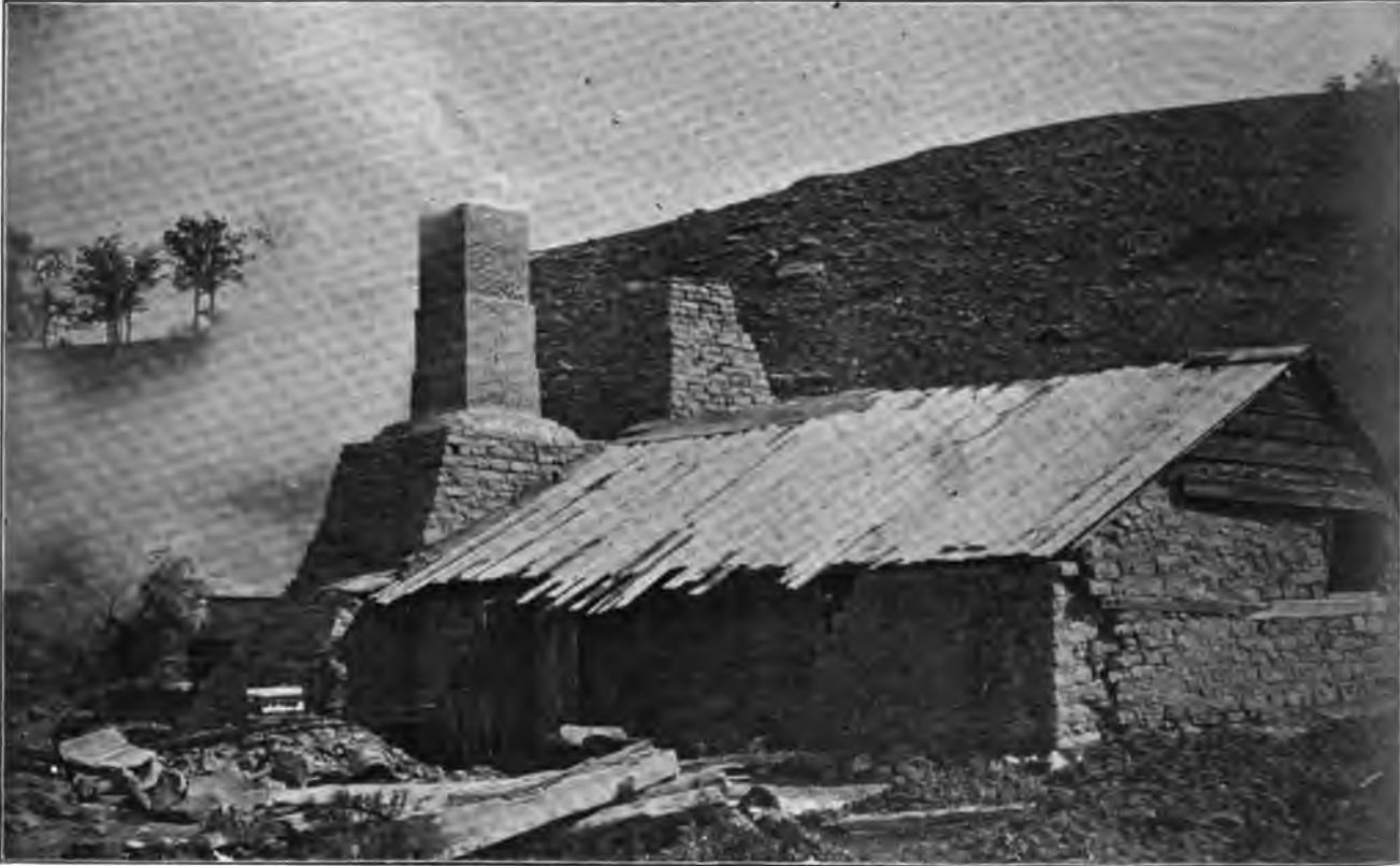
Water's lead furnace, near Dubuque, constructed in 1834. The first hearth lead furnace in Iowa and the second in America.
